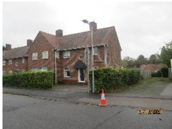
Principal elevation of 10 Midland Road
