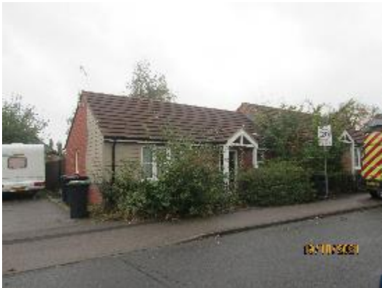
Principal elevation of 8 Midland Road
